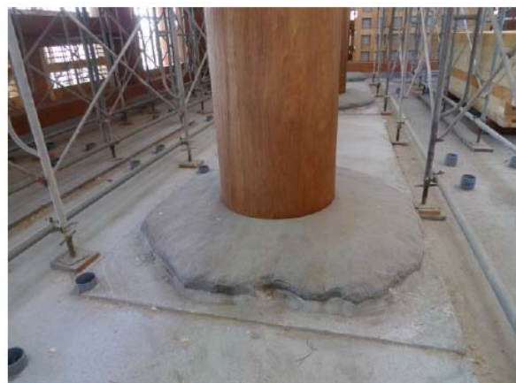
Figure 7 Kofuku-ji Central Golden Hall reconstruction site. The columns, 80 cm in diameter, in rows are from African Apa trees. Photograph by the author.
