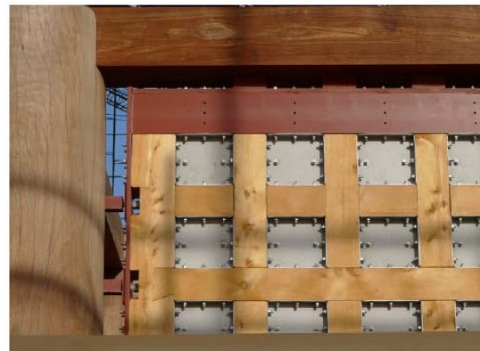
Figure 8 Anti-seismic stainless latticework in a wall of the Kofuku-ji Central Golden Hall. Photograph by the author.
