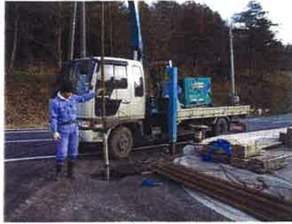
Installation of drawing pump
